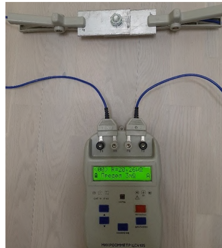
Fig. 5. Measuring the resistance of the contact connection
