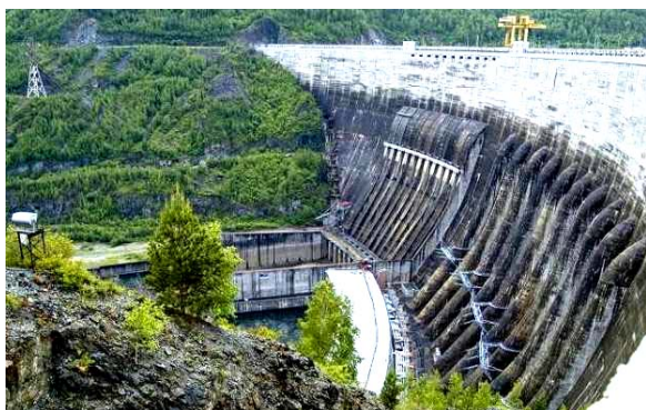
Fig. 9. General view of the largest in Russia Sayano-Shushenskaya HPP of dam type with power of 6400 MW (the Yenisei River) [4]
