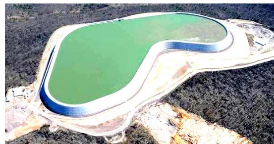
Fig. 10. Stunning general view from the height of the «bird's eye view» of the huge reinforced concrete reservoir at the top of the remote from the cities of the mountain range of the modern pumped storage power plant «Taum Sauk» (USA) [13]
