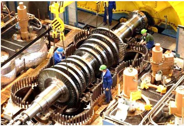
Fig. 4. Installation of a powerful domestic steam turbine ПТ-1000 (in the right side of the turbine axis, the body of the corresponding turbogenerator is visible) in the power plant hall of the NPP [9]
