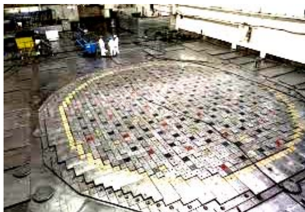
Fig. 7. General view of a powerful nuclear reactor of the RBMK-1000 type installed in the reactor plant of one of the 4 operated power units of the Chernobyl nuclear power plant (before the catastrophe in 1986) from its assembled of separate lead blocks of the upper protective cover [2, 9]
