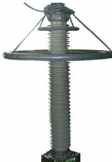
Fig. 11. A high-voltage divider class 220 kV for measuring the power quality indices (outdoor design)
