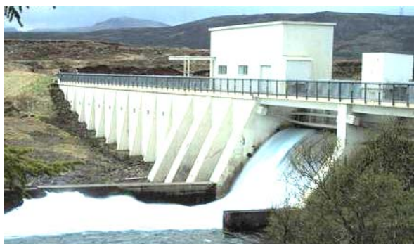
Fig. 28. General view of the dam and engine room of the domestic SHPP (2009, Ukraine) [30]
