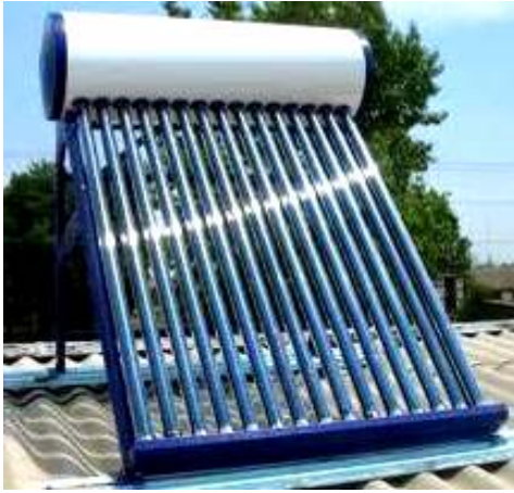
Fig. 10. General view of the solar collector at the photometric method of using the light flux of energy [3]
