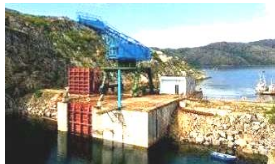
Fig. 26. General view of the TPP «Kislogubskaya» of power of 1.7 MW (1968, Sour lip, Kola Peninsula, Russia) [6]
