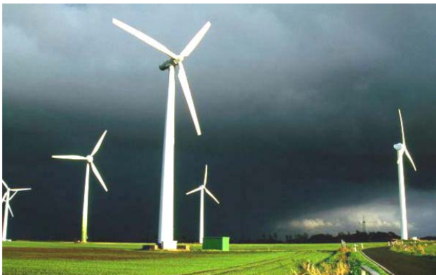
Fig. 1. General view of modern horizontal-axis three-bladed wind turbines installed, located on the flat coastal area up to 250 kW [10]
