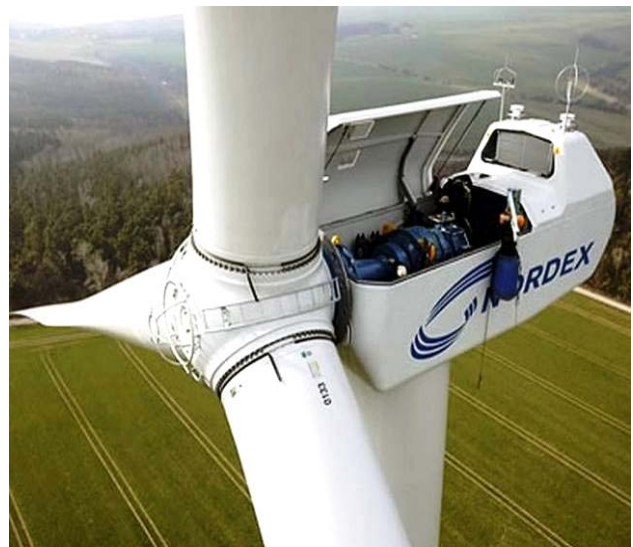
Fig. 4. The enlarged view of the turbine of modern horizontal-axis three-bladed wind turbines NORDEX marks the installed capacity of up to 1500 kW land-based during its maintenance at a height of about 70 m [11]
