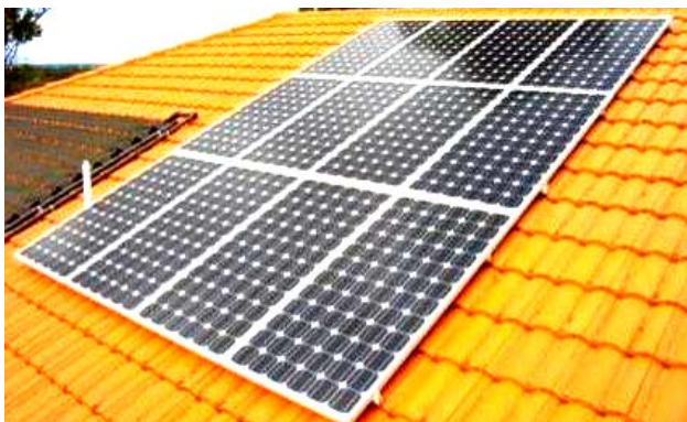
Fig. 12. External view of a rigidly fixed small solar panel mounted on the roof of the house [15]
