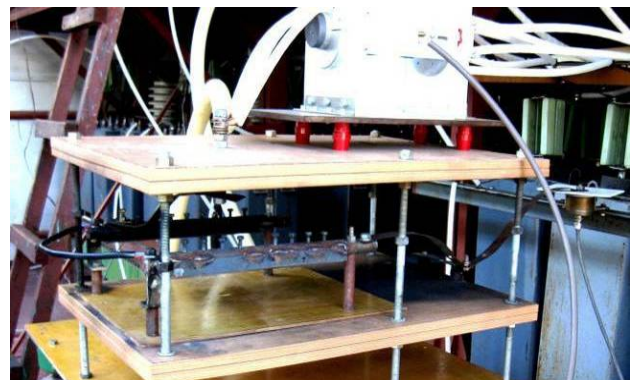
Fig. 13. View of the wire АППВНг2×6 with PVC insulation of the length of 0.5 m with its parallel electrodes connected to working table of the generator ГИТМ-10/350 with two aluminum cords of total section of S_1 \approx 12 \text{ mm}^2 to exposure by the pulse current 15/335 \mu\text{s} of the artificial lightning of amplitude I_{mL} \approx 83.8 \text{ кА} (on the right the measurement shunt ШК-300 [7, 10] included in the high-current discharge circuit of the generator is clearly shown)
