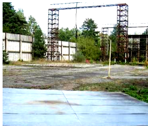
Fig. 4. General view of the high-voltage aerial DEDS «tip-plane» ( l_{min} = 1,5 m), in which an ohmic voltage divider of the OPN-2.5 type for a nominal pulse voltage of \pm 2,5 MV with division factor equal to K_d \approx 53650 is connected to the potential upper steel rod electrode pointed at the lower edge ( r \approx 3 mm) with radius r_0 \approx 15 mm, located in the center of its grounded lower flat electrode made of galvanized steel with dimensions of 5 \text{ m} \times 5 \text{ m}
