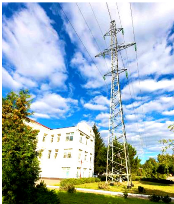
Fig. 2. Residential building closed to double-circuit power line
