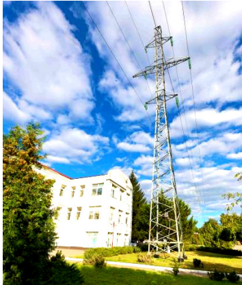
Fig. 2. Residential building closed to double-circuit power line
