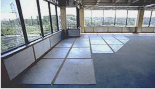
Fig. 1. The room located near power lines
