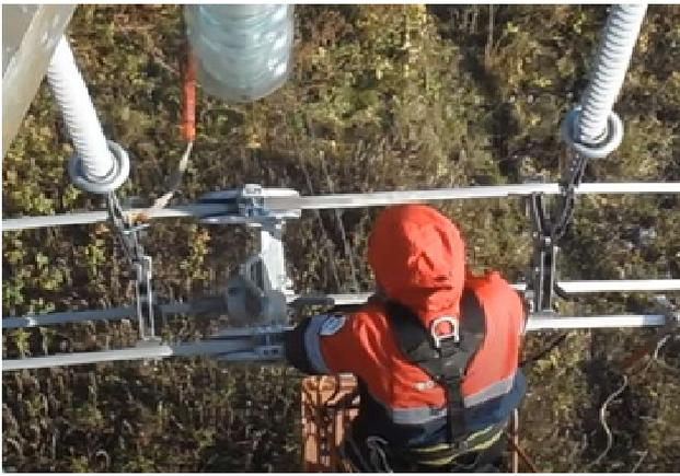
Fig. 1. Execution of repair works by NPC «Ukrenergo» on the 330 kV power line under voltage
