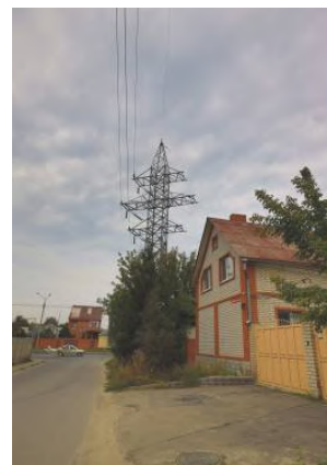
Fig. 1. Location of a residential building near overhead power transmission lines
