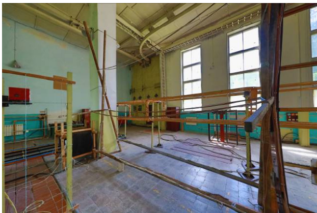
Fig. 6. Location of three compensating windings of experimental plant of system of active shielding
