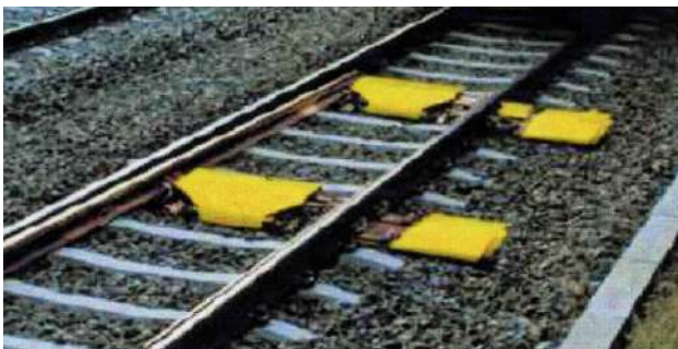
Fig. 1. General view of the EBI Switch 2000 turnout
