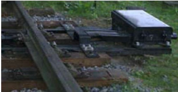
Fig. 3. External view of the SP-6m turnout
