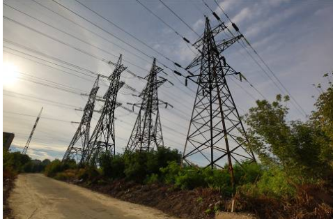
Fig. 1. Location of a group of high voltage power lines
