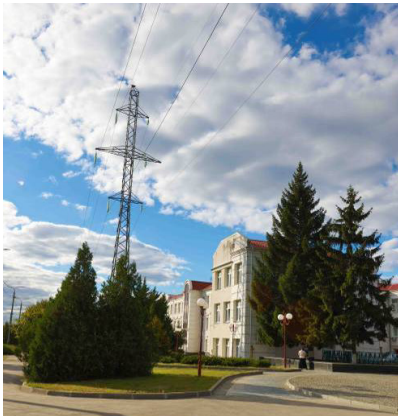
Fig. 2. Residential building closed to double-circuit power line
