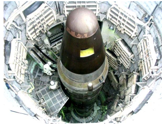
Fig. 5. General view of the ML with the Soviet P-36M type ICBM installed in it (military index 15A14, SS-18 «Satan») during maintenance of the missile by military personnel from folding platforms [14]
