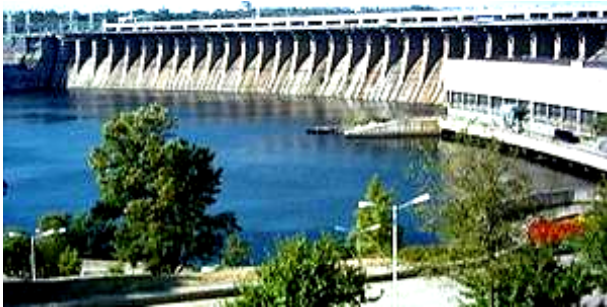
Fig. 12. Modern general view of the Dneprovskaya HPP [15]
