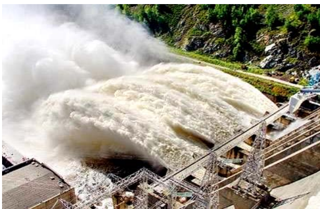
Fig. 1. Impressive and mesmerizing our imagination the power of river water discharged through open water lines in a reinforced concrete dam from an artificially created reservoir of modern HPP [2]
