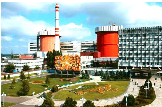
Fig. 11. General view of the fragment of the South-Ukrainian NPP with the total installed power of 3000 MW (Yuzhnoukrainsk, Mykolayiv region, Ukraine) [17]
