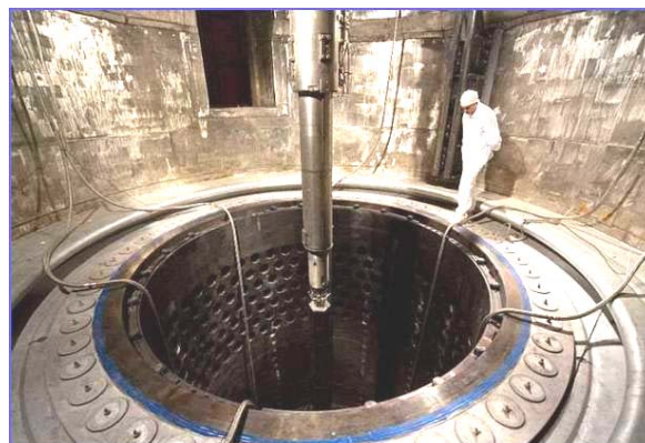
Fig. 9. Loading of fresh fuel (fuel assemblies) into a powerful water-water nuclear reactor of the WWER-1000 type (the upper hermetic protective cover of the reactor was removed) [2, 9]
