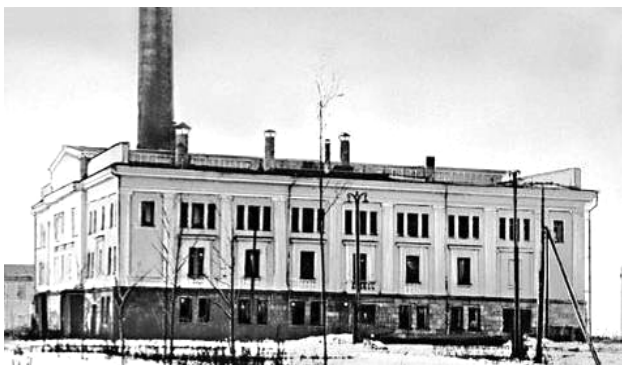
Fig. 1. General view of the main building of the world's first pilot industrial Obninsk NPP with installed power of 5 MW (Obninsk, Kaluga region, RF, 1954) [7]
