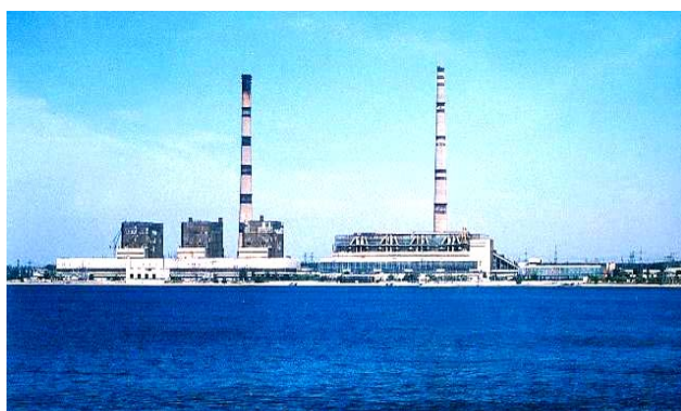
Fig. 6. General view of the Uglegorskaya TPP with installed power of 3,600 MW with a nearby lake-cooler [4]
