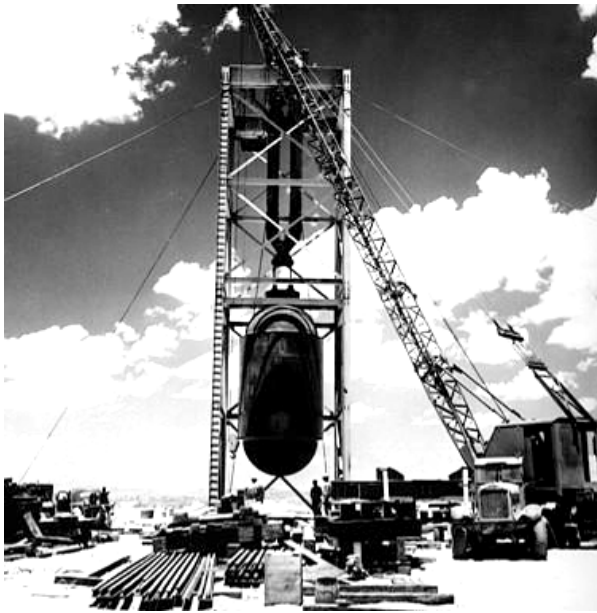
Fig. 3. The general view of the epicenter of a future nuclear explosion with a steel tower up to 30 m high, on top of which the first American plutonium atomic bomb «Trinity» (US military probe in the Alamogordo Desert, New Mexico) was moved there with the help of lifting equipment, July 15, 1945) [7]
