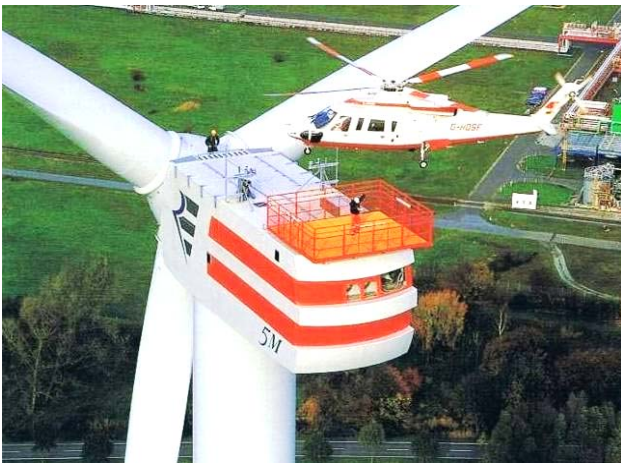
Fig. 6. Moment of involving maintenance of the helicopter crew at a height of 80 m land-based Norwegian horizontal axis three-bladed wind turbine with the largest installed capacity of up to 5000 kW [11]
