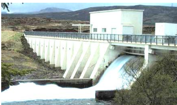
Fig. 28. General view of the dam and engine room of the domestic SHPP (2009, Ukraine) [30]
